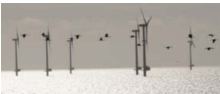
Picture 12. Cranes passing on the side of the wind turbines at Utgrunden.
