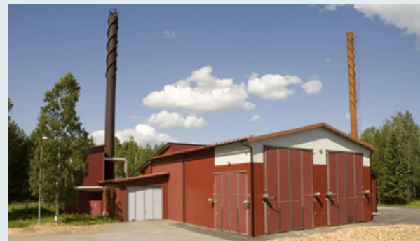
Photo: Bollnäs Energi
